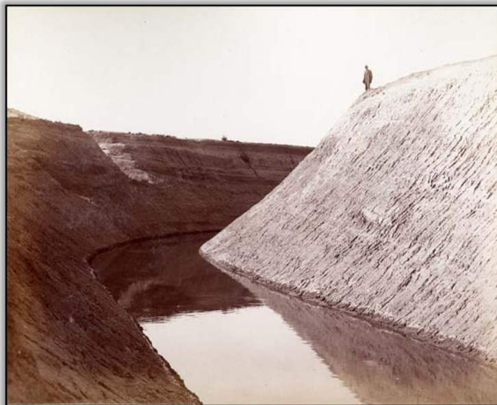
Deep cut irrigation canal "Pot Hole Division" near Magrath circa 1890 - 1905. Photo credit Galt Museum & Archives.
